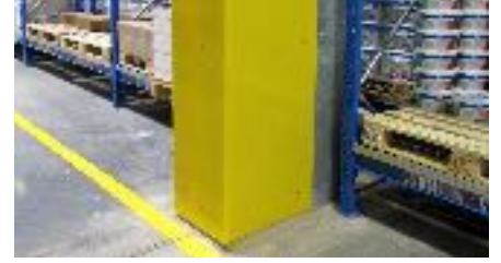
Collision protection for cement pile
