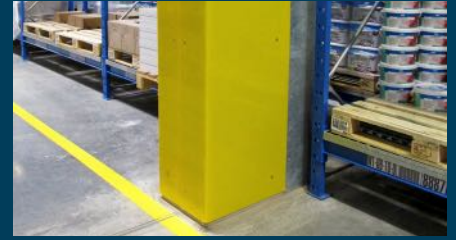
Collision protection for cement pile
